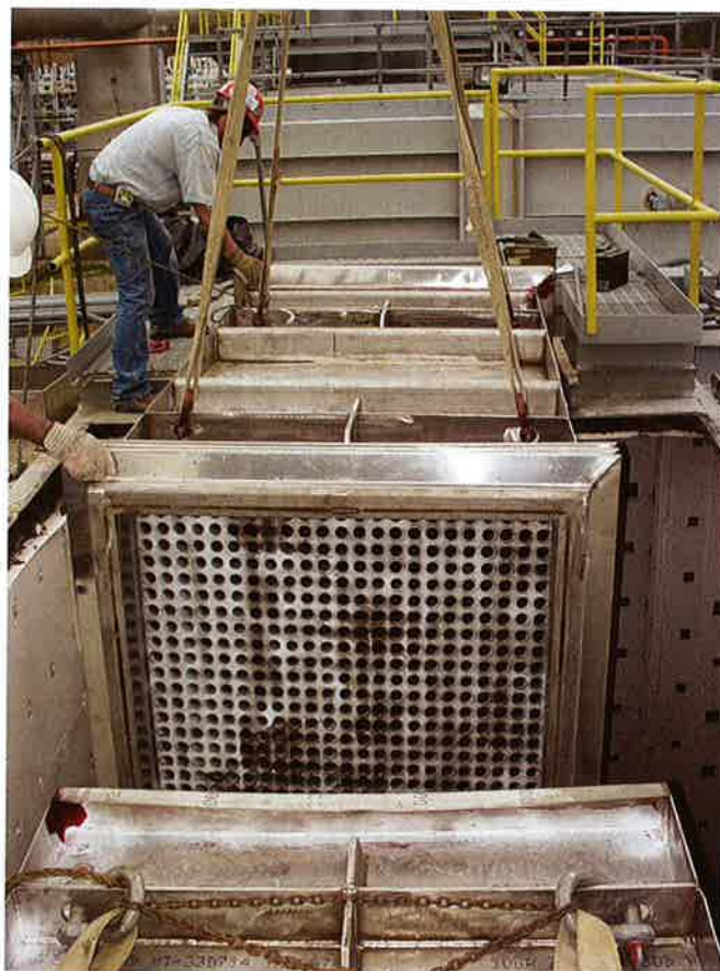
Maximizing internal thermal energy recover. Metal heat exchanger replacement.
